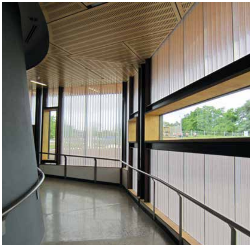
Edificio Australian Centre of Excellence Eureka Stockade en Victoria (Australia) Arquitectura: William Boag Allen Architects.
